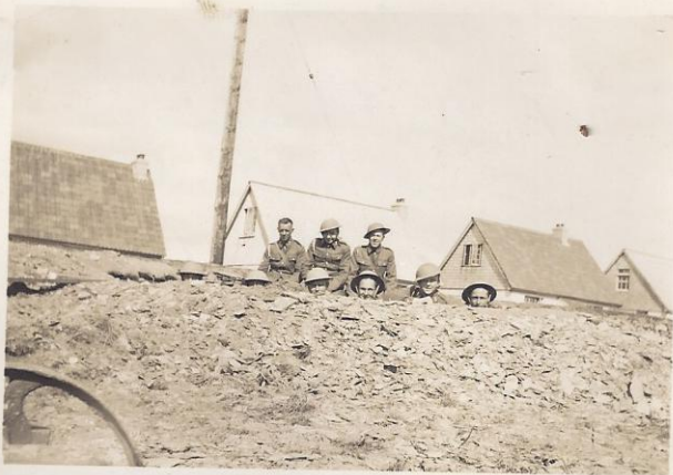
Some of our P.A.D - Trenches -
