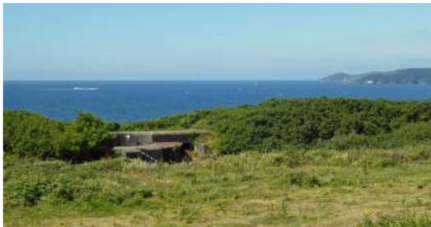
Figure 6 Seaward view from the Lentney site. The concrete building is part of the battery. © David Pinder
