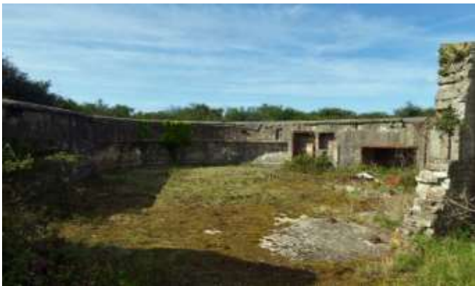
Figure 20 View into a Renney Battery gunpit from the rear
