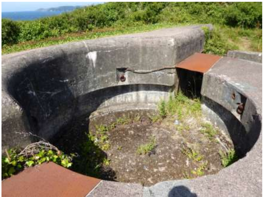
Figure 12 Above: Rear view of Lentney Battery; below: 6" gunpit at Lentney ©David Pinder
