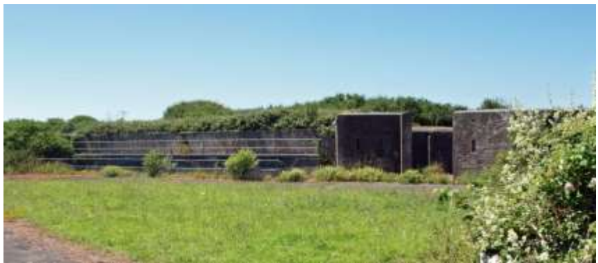
Figure 15 Rear view of Renney Battery. One of the gunpit entrances is to the right of the large black blast wall. © David Pinder
