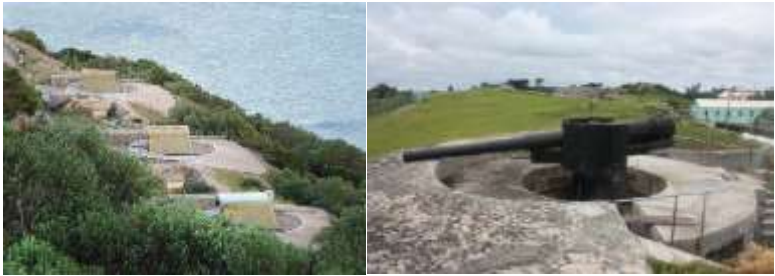
Figure 18 Two contrasted approaches to 6" gun crew protection
