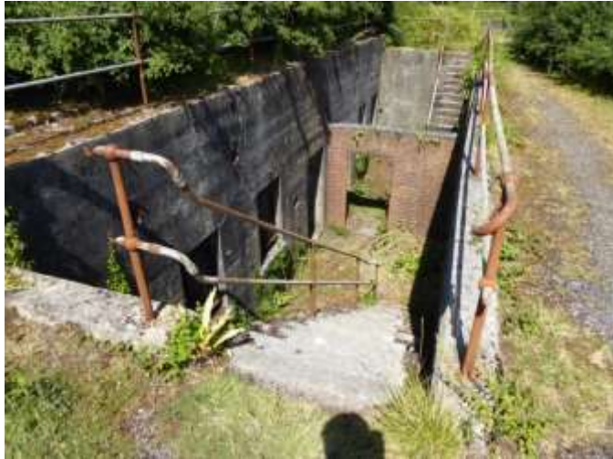
Figure 14 Steps down to one of Lentney Battery's magazines © David Pinder
