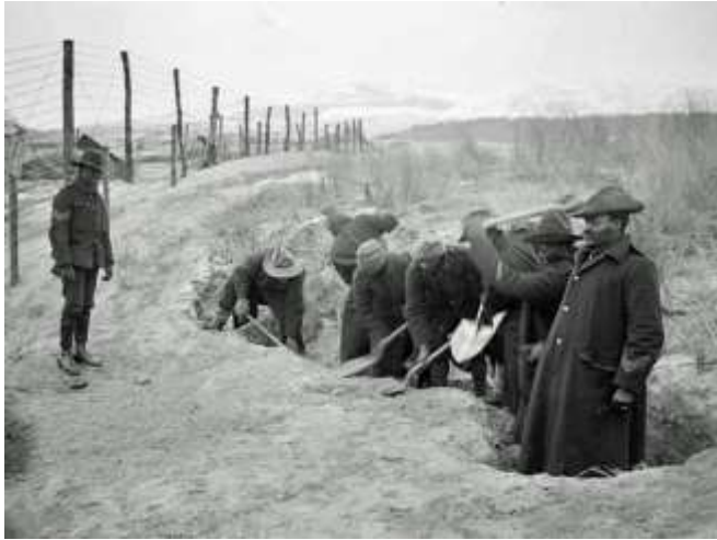
Figure 18 SANLC members trench digging. The camp fence can be seen in the background.
